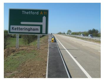
The quality of the existing concrete road surface was still good with little or no surface preparation required, initial trials were done to convince the contractor as to there suitability for the project, they were very sceptical about the kerbs ability to with stand the rolling of the asphalt pavement behind the kerb, but later admitted to being surprised by the kerbs performance.
