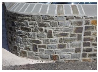
Rather than using traditional copings to complete the wall, sawn and flamed pennant slabs were used installed at an angle to create a "Bishops Hat" coping detail, the flame finish applied to the pennant slabs gives a riven type finish. The whole wall has blended in very well and already looks like part of the historic town
