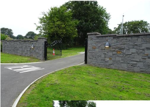
With the construction of the new Nantgarw Cemetery, Caerphilly County Borough Council, were looking to a traditional Welsh stone laid in a coursed walling design, courses of 65/140 & 215mm were chosen in random lengths, the two smaller courses being split face and the 215mm flamed. The gate post pillars were built incorporating 450 x 225 x 100 dressed quoins, 675mm wide x random length (500-900mm) x 100mm copings, and large 675 x 675 x 100 pillar caps all with flamed top and sides
